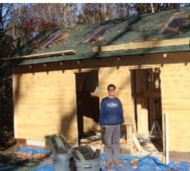
Junior Bathroom is being remodeled.
