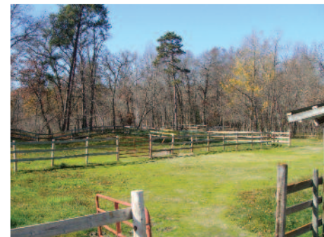
Lots of corral fence repair and replacement.
