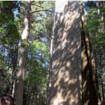
The Climbing Wall has a new layer of wood chips and awaits the new overhang to be installed next spring.
