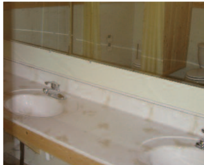
New bathroom in Orioles Cabin.
