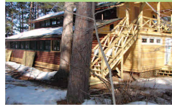
Nutcracker remodeling almost complete.
