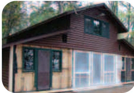
Construction on Nutcracker remodeling lake side.
