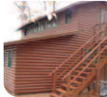
Rangers cabin gets new paint job.
