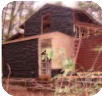
Construction on Nutcracker remodeling back side of cabin.
