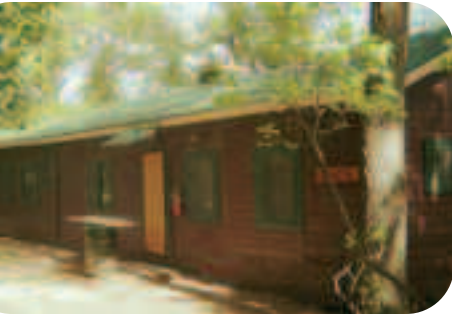
Apache Cabin get an upgrade new roof and remodeled bathroom.
