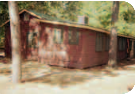
Apache Cabin lake side upgrade.
