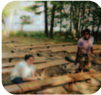
Chapel area cleaned and benches sanded filled and painted ready for 2008.
