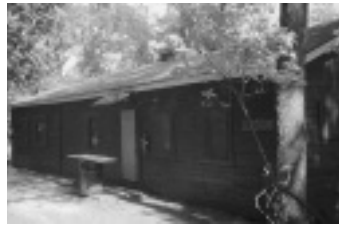
Apache Cabin gets an upgrade, new roof and remodeled bathroom.
