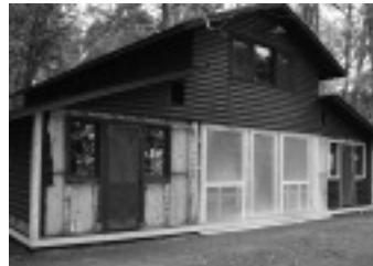
Construction on Nutcracker remodeling lake side.
