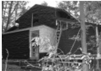
Construction on Nutcracker remodeling back side of cabin.
