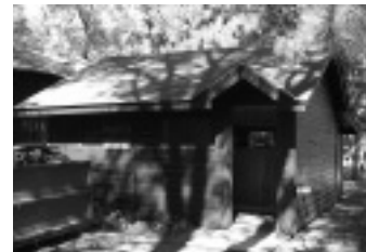
Zorba gets remodeled and a new roof too.
