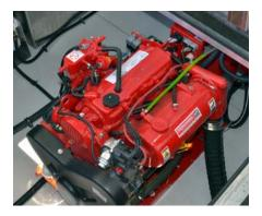
CAUTION: The blower must be used at least 5 minutes before starting the generator located below deck, to clear any fumes that may have collected.
